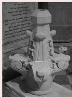
*Above: The new finial stone prior to installation. Left: Elevations of the spire showing stone to be replaced.*
